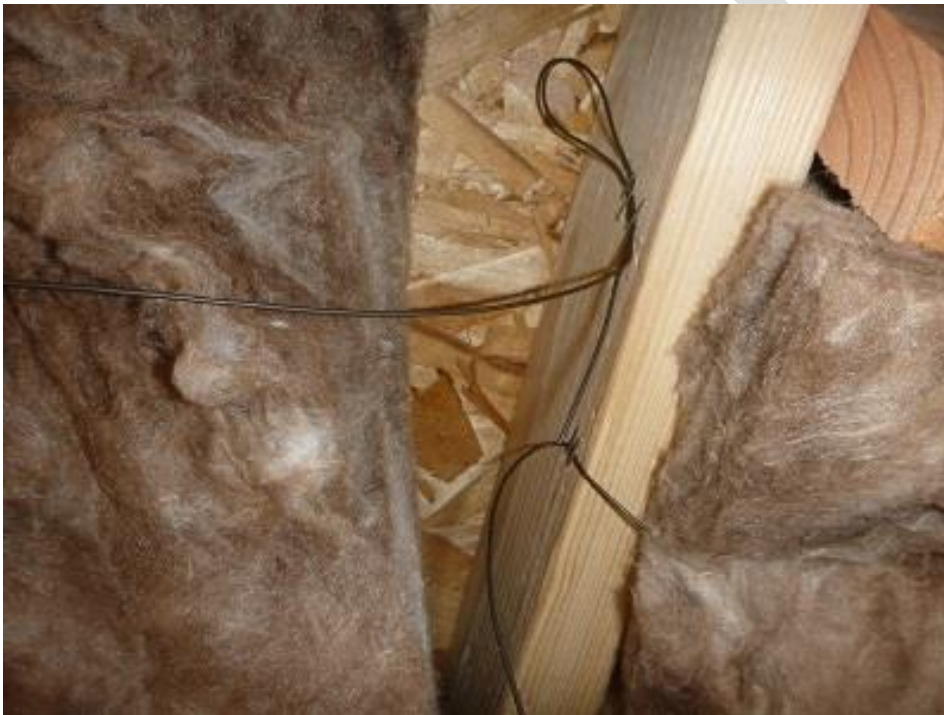
Figure 3: Example batt cabling securement method (insulation manually pulled back).
