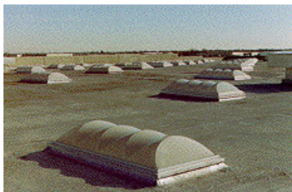
Figure 5: Compound parabolic skylight
