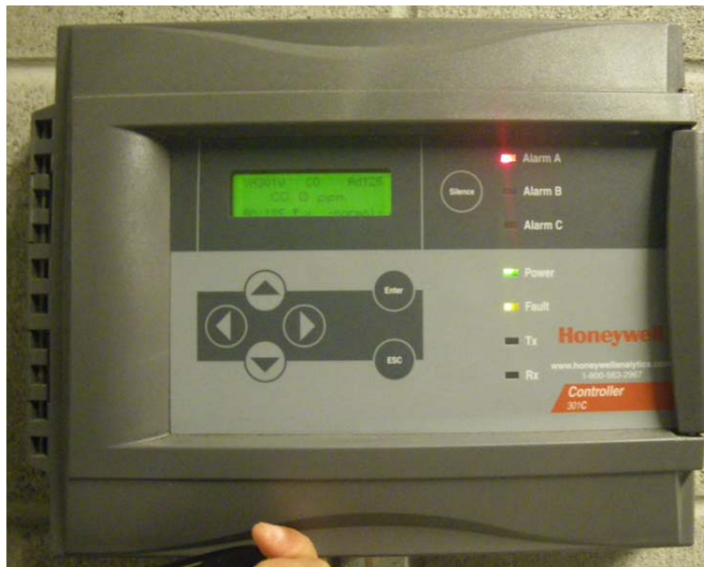
Figure 19. Typical CO sensor in Garage C
