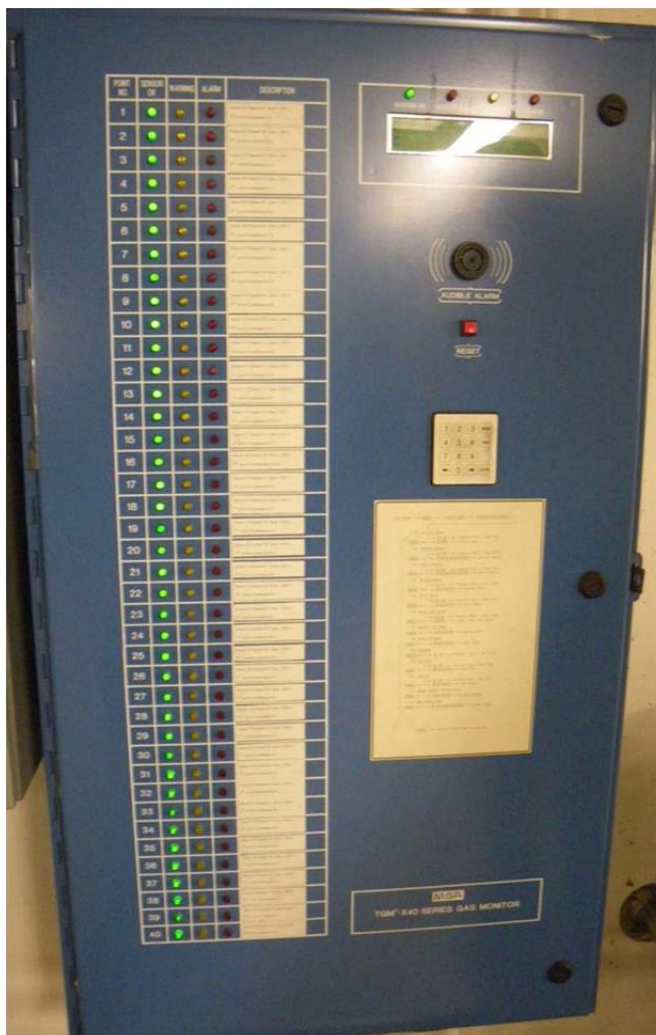
Figure 17. Sensor control panel in Garage B
