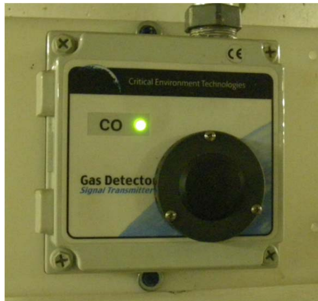
Figure 16. Typical CO sensor in Garage A
