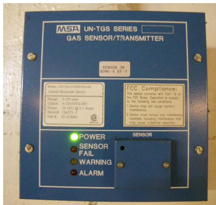
Figure 18. Typical CO sensor in Garage B
