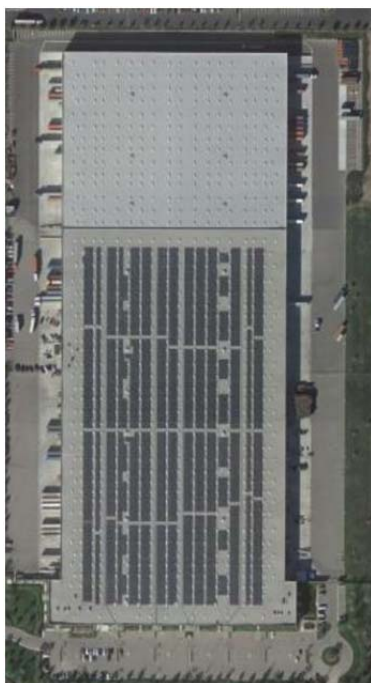
b. Warehouse with PV system
