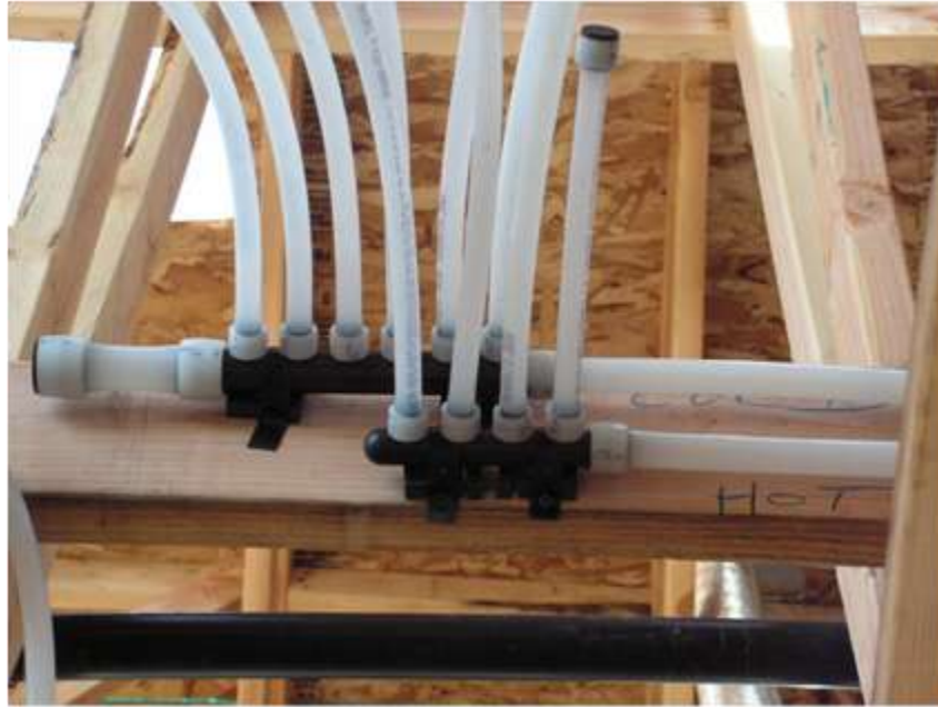
Figure 6: Installed Mini-Manifolds
