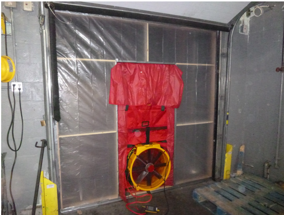
Figure 2: Dock door air leakage test apparatus.
