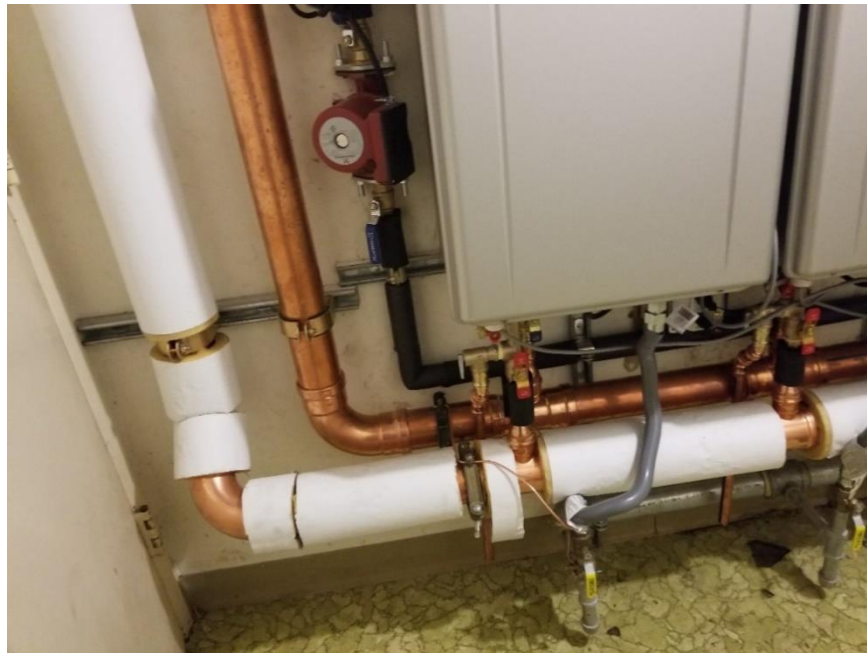
Figure 11: Uninsulated fittings and valves.
