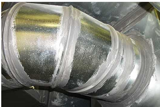
Figure 21: Duct with mastic applied.
