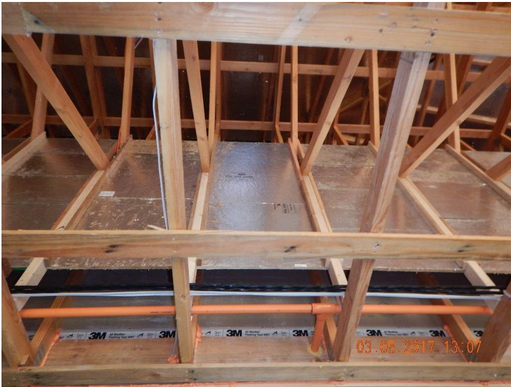
FIGURE 3. CONDITIONED MECHANICAL SPACE UNDER CONSTRUCTION (FROM BELOW).
