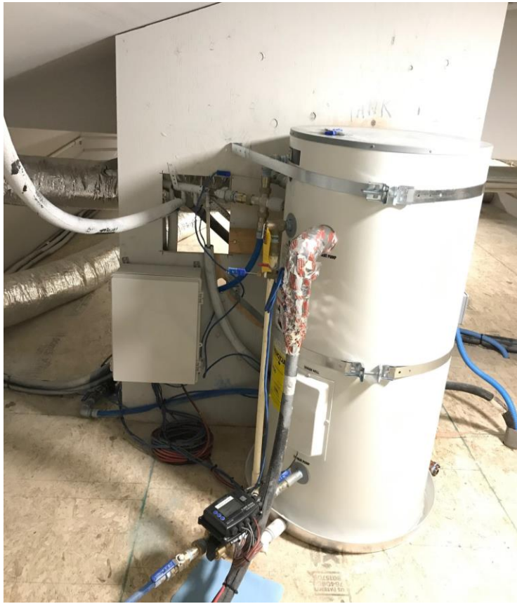
FIGURE 4. HPWH STORAGE TANK WITH FLOW METER AND THERMOCOUPLES INSTALLED.
