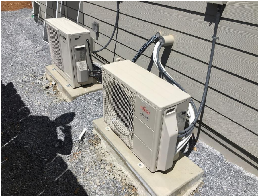
FIGURE 5. HPWH OUTDOOR UNIT (ON LEFT).
