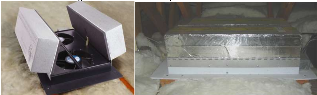
Figure 2: Insulated and Dampered Whole House Fan
