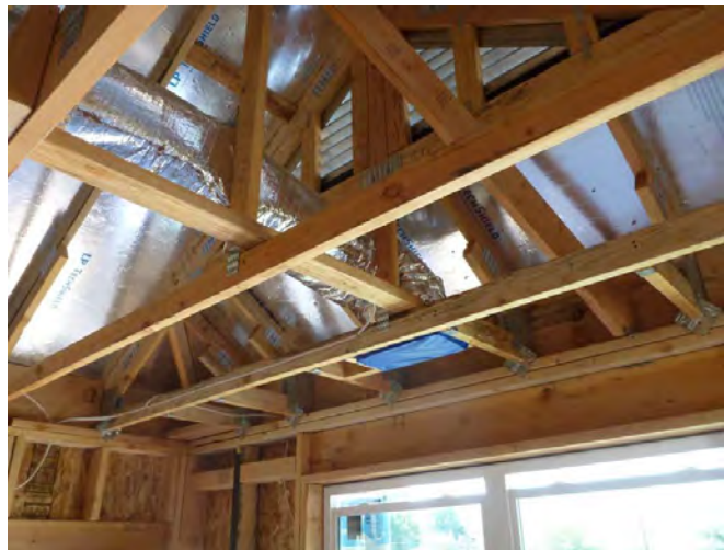
Figure 17: Below deck unfaced fiberglass batts and blown-in fiberglass on the ceiling floor.
