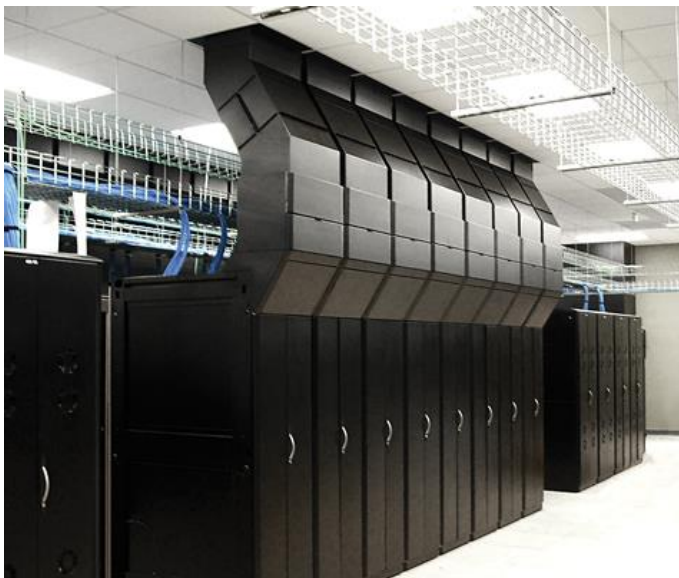
Figure 7. Example return air chimney and enclosed server rack product.
