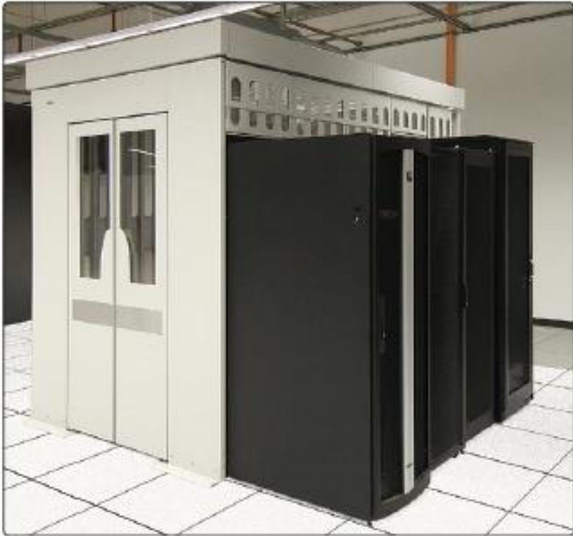
Figure 22. Example Containment System – Standard Hot Aisle Enclosure
