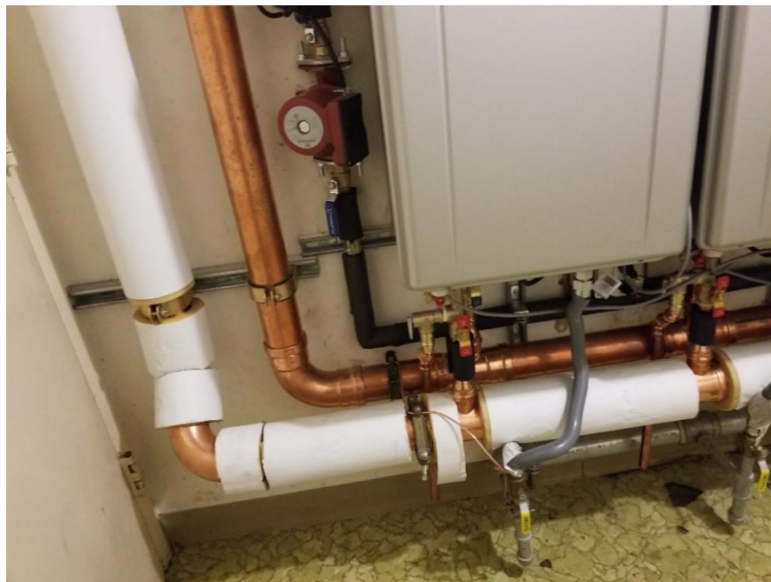
Figure 11: Uninsulated fittings and valves.
