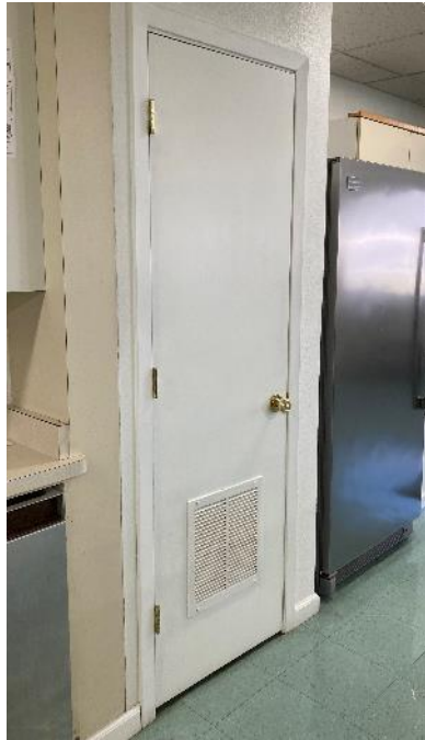
Figure 42: DHW closet door with lower grilles from a small commercial kitchen in Woodland, CA.
