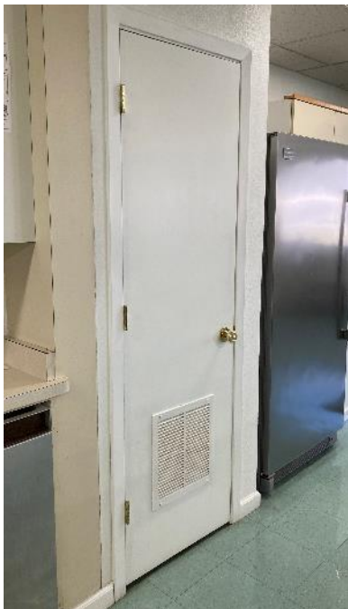
Figure 45: DHW closet door with lower grilles from a small commercial kitchen in Woodland, CA.
