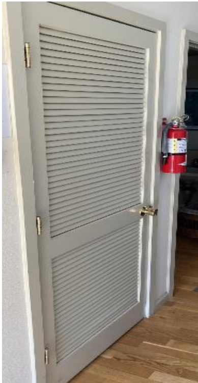
Figure 21: Fully louvered door.
