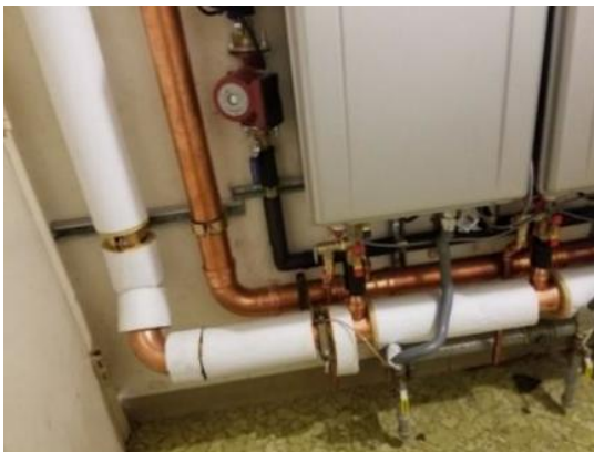
Figure 2: Field observation punch list photo showing missing pipe insulation.
