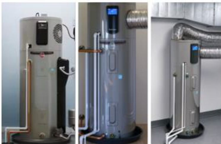
Figure 2: Example of a HPWH with no ducts (left), one duct (center) and two ducts (right) also known as fully ducted.
